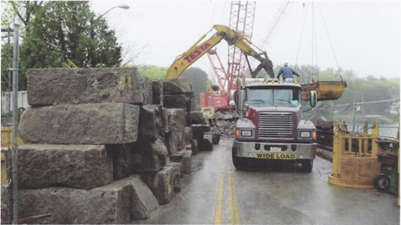
Longfellow Bridge rehabilitation and expansion project May 16, 2014 6:00 PM CDT
