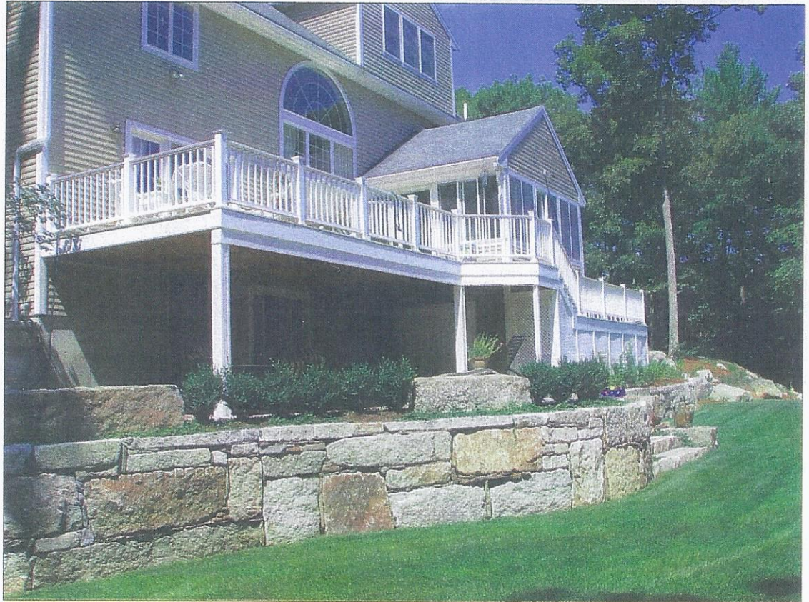
Olde New England Granite supplied the reclaimed granite block and cap material to form this beautiful and functional retaining wall and steps.
